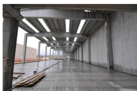
**Fig. 1 Typical RC precast building system**
